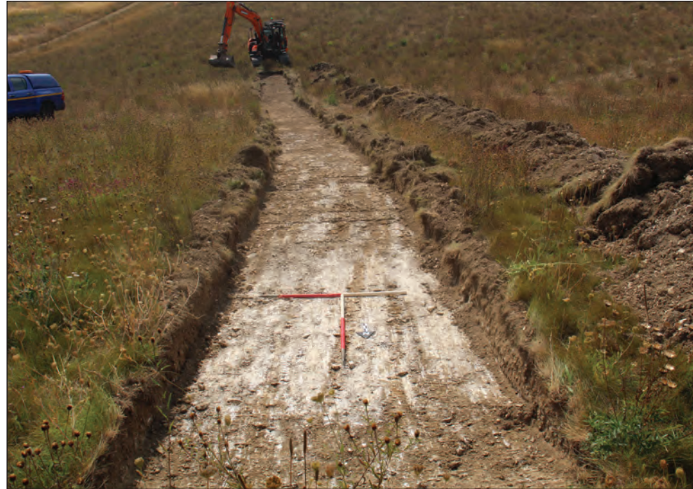
Trench 79, looking south (1m scales)
